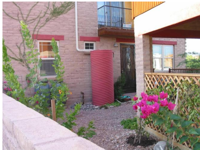
This simple cistern was made with corrugated steel drainpipe and can hold up to 400 gallons. Photo by Scott Calhoun.
