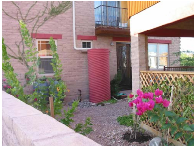
This simple cistern was made with corrugated steel drainpipe and can hold up to 400 gallons. Photo by Scott Calhoun.
