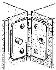
To prevent this, remove two opposing screws from each leaf of the hinge. Screw a lag bolt into the jamb, sawing off the head. Or use a headless nail, leaving 1/2 inch of the nail or bolt protruding. Drill out the opposite hole in the jamb leaf. Do this to both top and bottom hinges. When the door is closed the hinge pins may be removed, but the door will remain firmly in place.
