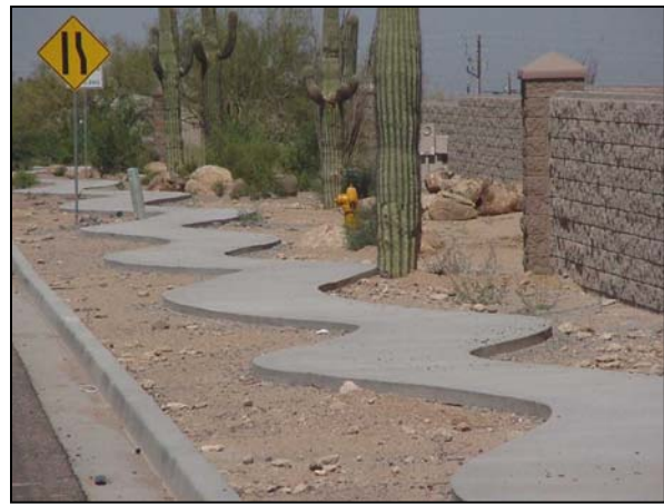
Sidewalks that meander unnecessarily are less pedestrian friendly, especially for the elderly and those with disabilities.
