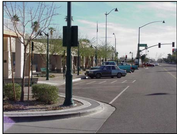
Angle parking in a well-designed streetscape.
