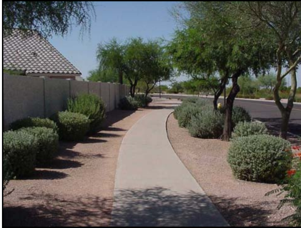
A detached sidewalk with trees and shrubs buffers pedestrians from street traffic
