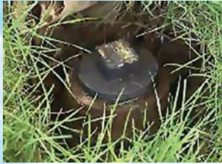
Sewer cleanouts can often get covered by landscaping.
