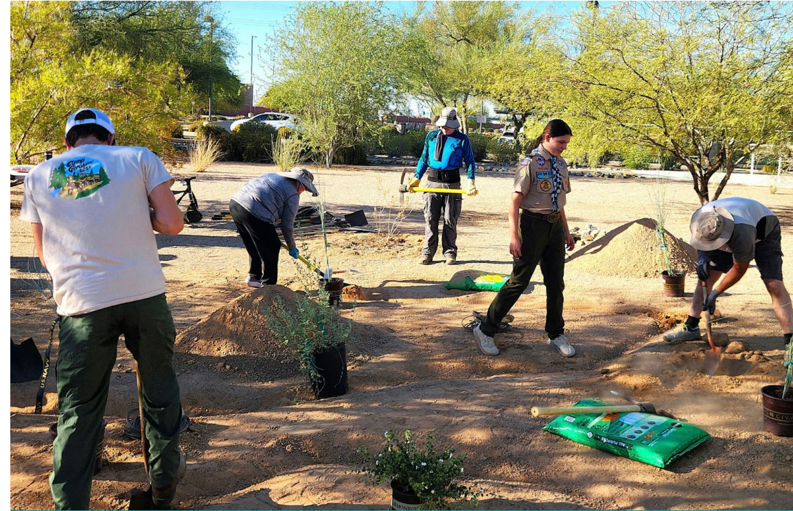
BSA Troop 3030 constructing a Monarch Waystation within the Monarch Haven & Reading Sanctuary at the Red Mountain Library
