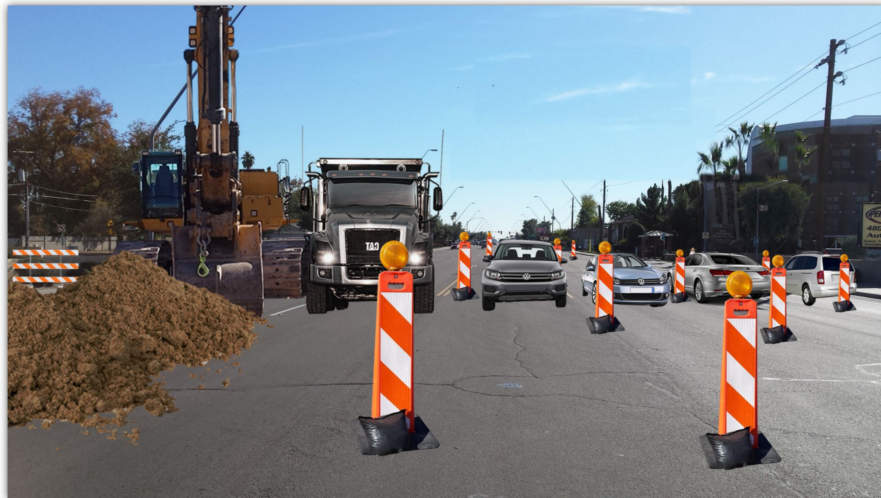
Typical traffic control during construction
