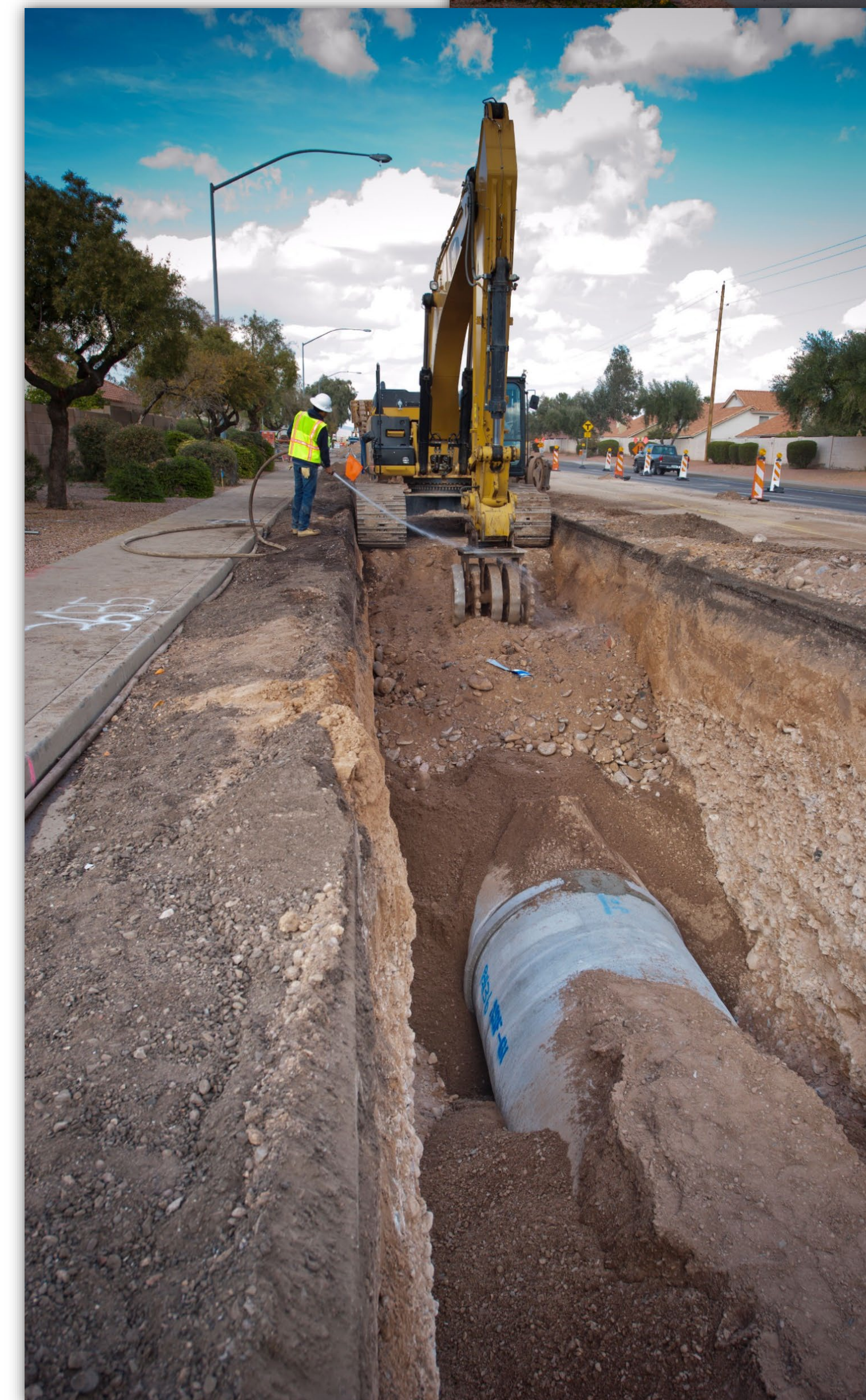
Pipe staged in roadway and excavation of trench
